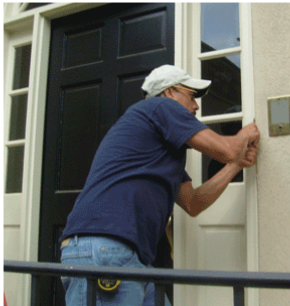
3. Cut Exterior seams with razor knife
