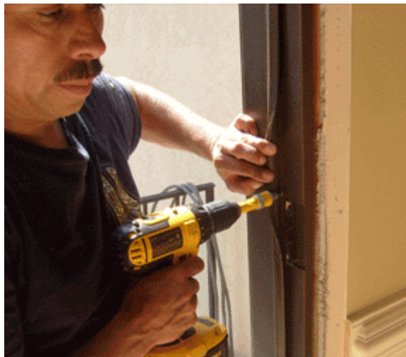
8. Temporarily position new doorframe into the old opening. Using temporary shims as a backer, Install a 3" drywall screw behind the middle hinge hidden under the weather-stripping. This will secure the frame while installing the doors, yet still allow for adjustment of the frame. Using the doors themselves in the frame is the best way to be sure the doors are fitting properly.
