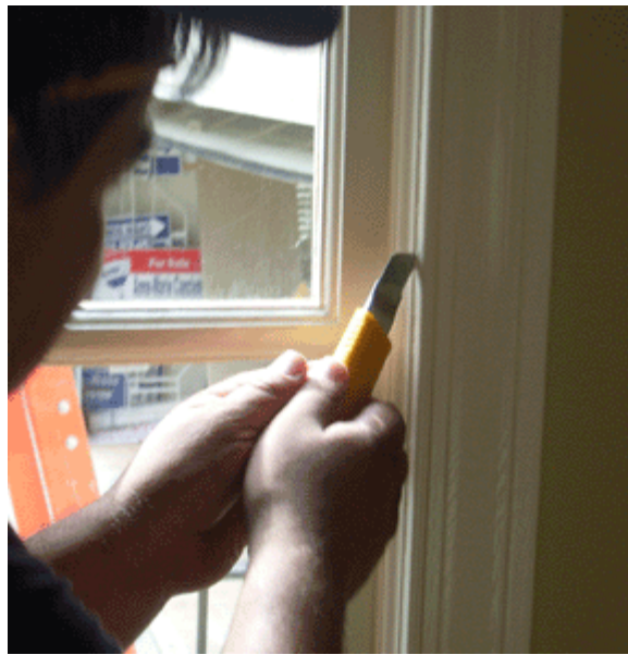
2. Cut interior trim seams with a razor knife
