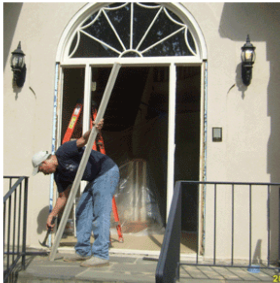
5. Remove Exterior Casing
