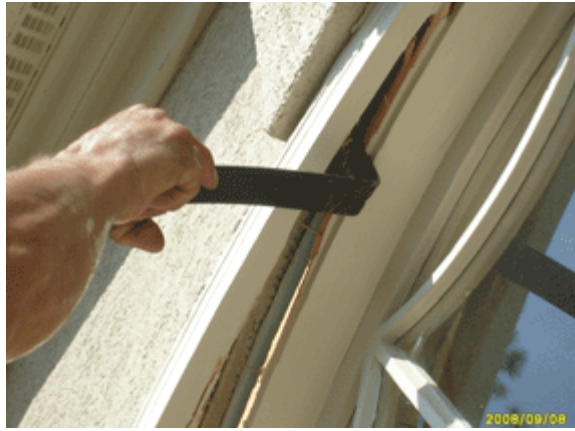
Slowly remove casing to avoid damage to the stucco or other wall surface
