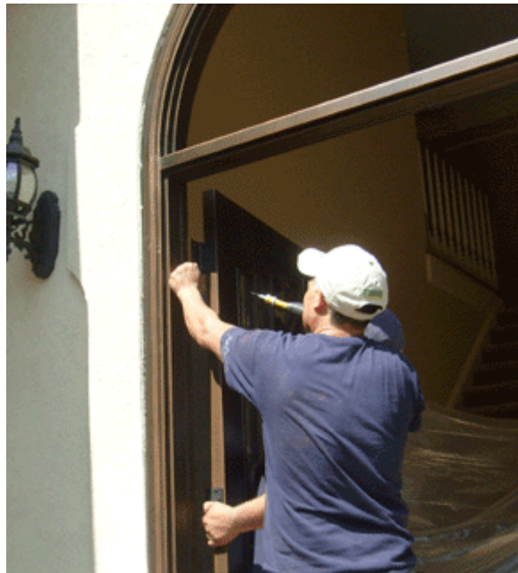
8. Temporarily position new doorframe into the old opening. Using temporary shims as a backer, Install a 3" drywall screw behind the middle hinge hidden under the weather-stripping. This will secure the frame while installing the doors, yet still allow for adjustment of the frame. Using the doors themselves in the frame is the best way to be sure the doors are fitting properly.
