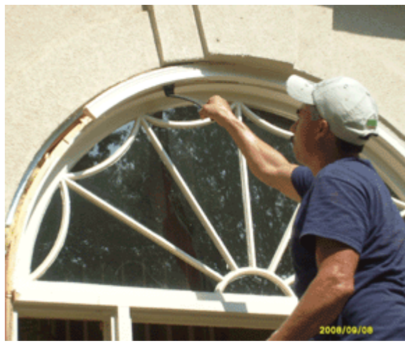
Slowly remove casing to avoid damage to the stucco or other wall surface
